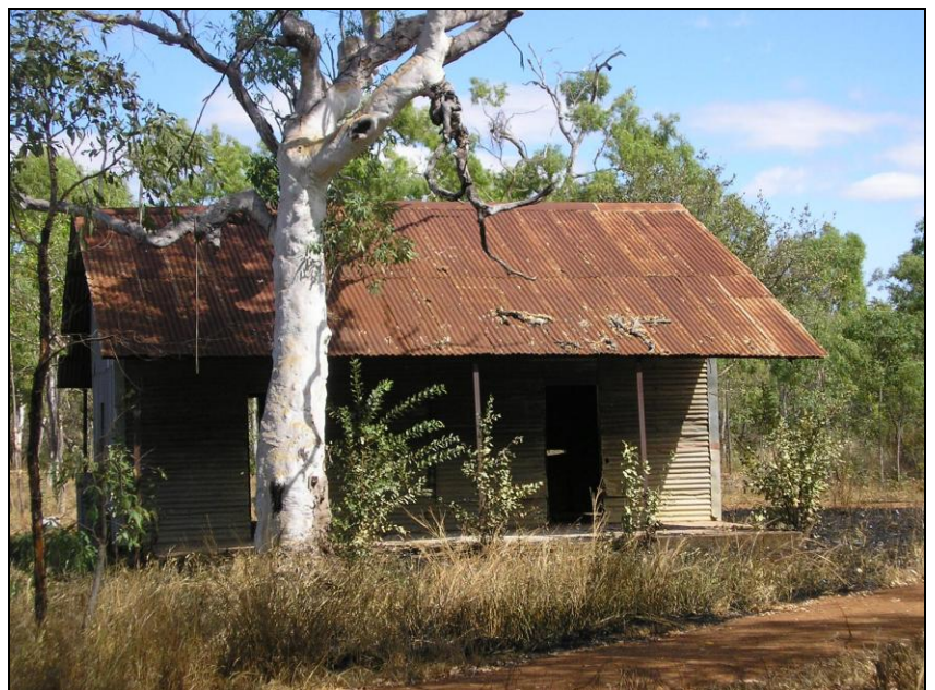
Old Roper Bar Police Station
