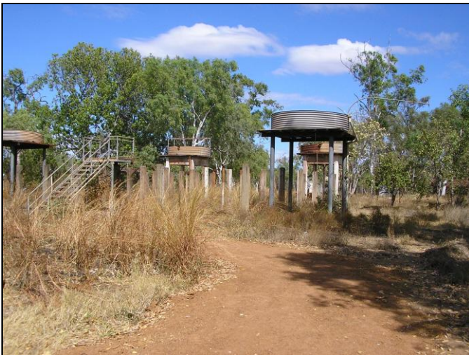
Old Roper Bar Police Station elevated water tanks
