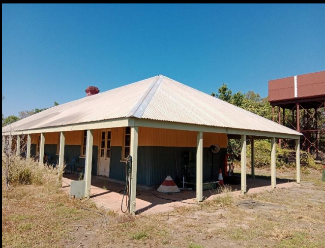
Adelaide River Railway Station showing the elevated water tank in the background
