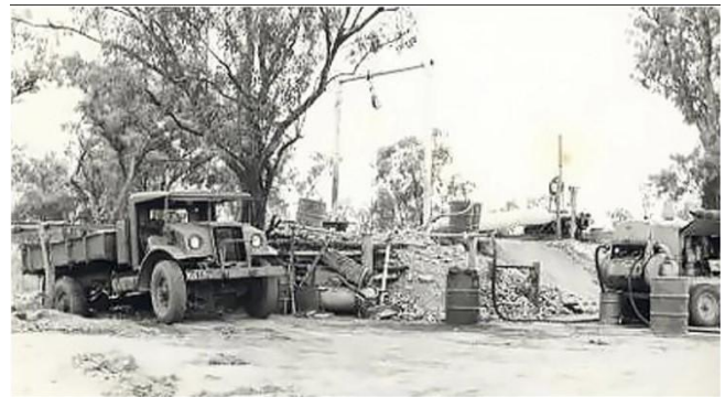
Unknown photographer, Early Drilling at McArthur River Mine, c1930s
