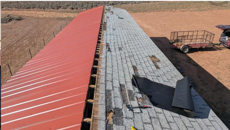
Before and Almost-after Roof
