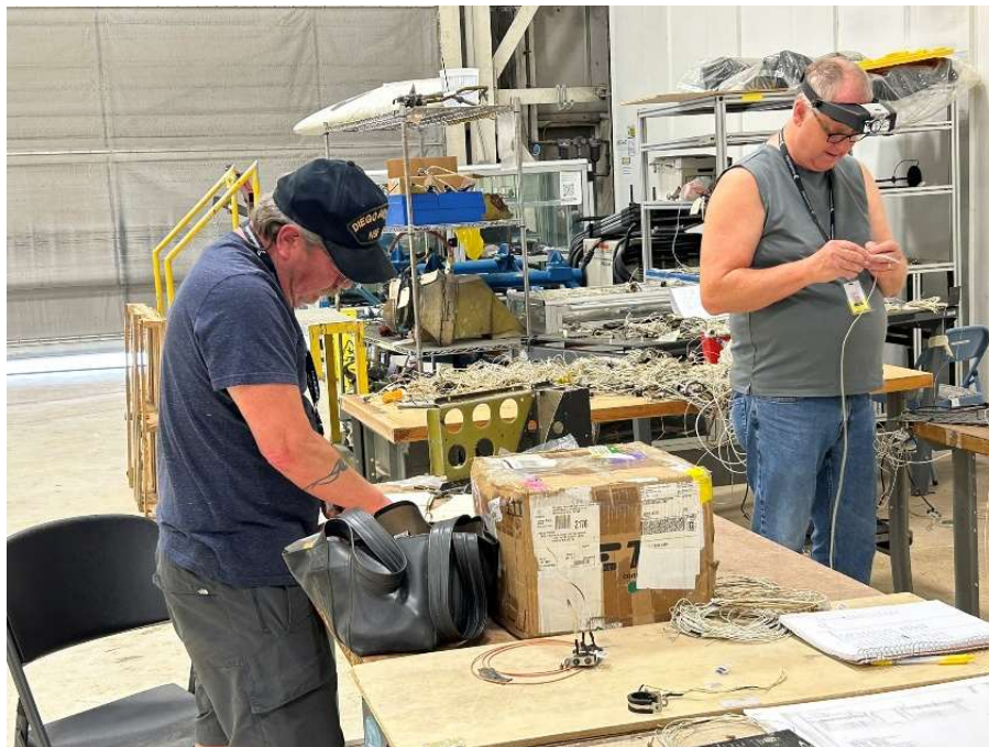
Bud Ledom, Rob Bielman - Working on Wiring
