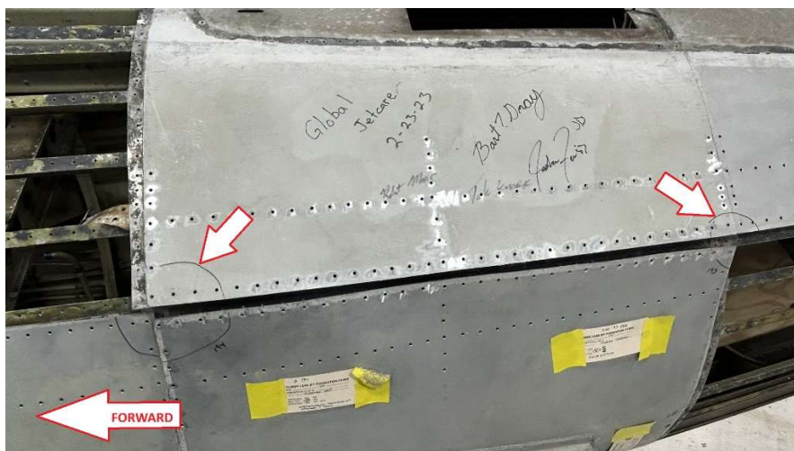
Skins Being Removed – Arrows at Areas of Concern
