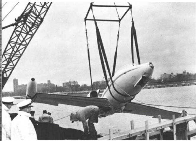
23-061 being lifted out of Lake Michigan
