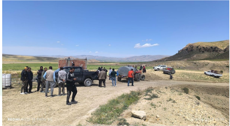
Repair of community water infrastructure by PhosCo
