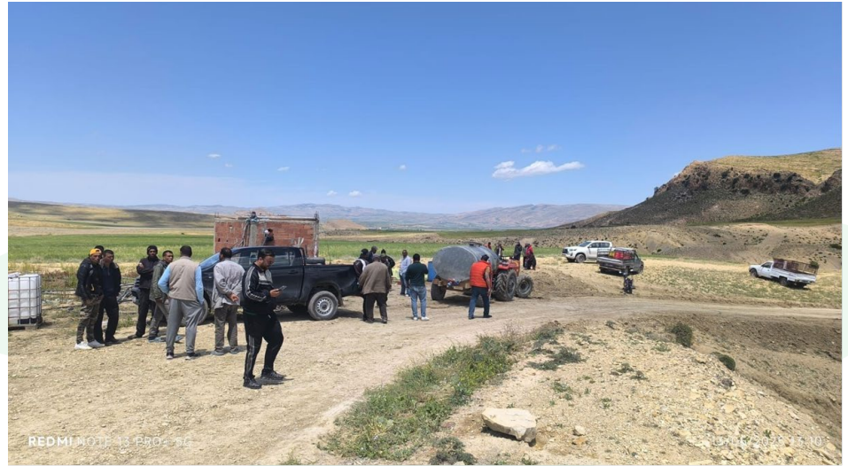
Repair of community water infrastructure by PhosCo
