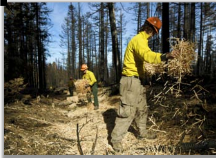
Image 8 Spreading mulch to reduce erosion
