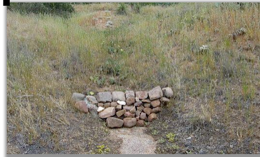
Image 7 A checkdam stabilizes soil behind it
