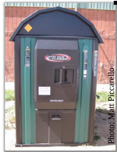
Image 3. Cordwood boiler installed outside of transfer station
