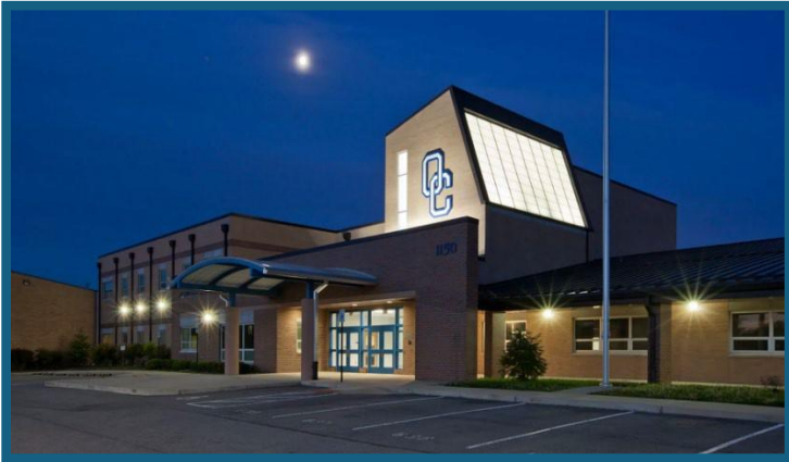
Oldham County High School
