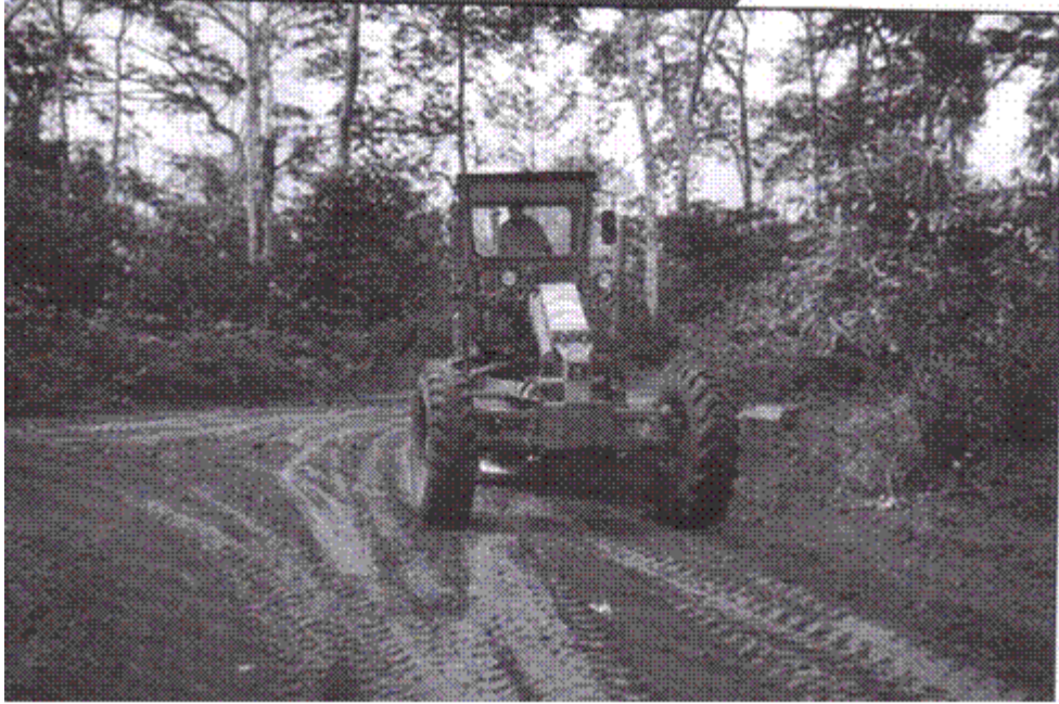
Council Caterpillar Maintaining the Road network During the Rainy Season
