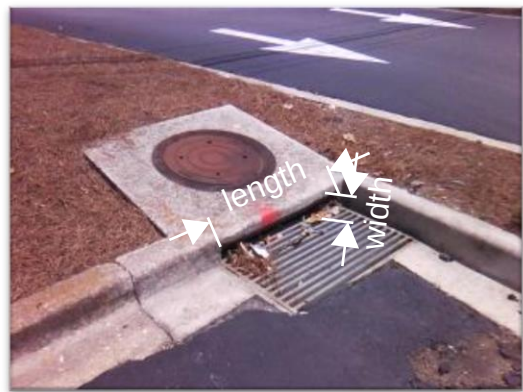
Combination (with Manhole Access)
