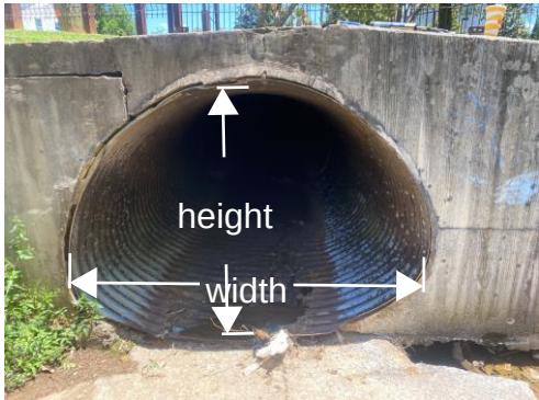
Pipe Arch Culvert
