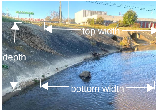
Ditch (sides are not earthen)
