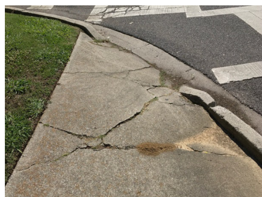
FIGURE 4: NON-COMPLIANT CURB RAMP (DUE TO EXCESSIVE SLOPES, SEVERE DETERIORATION, AND NO DETECTABLE WARNING SURFACES)
