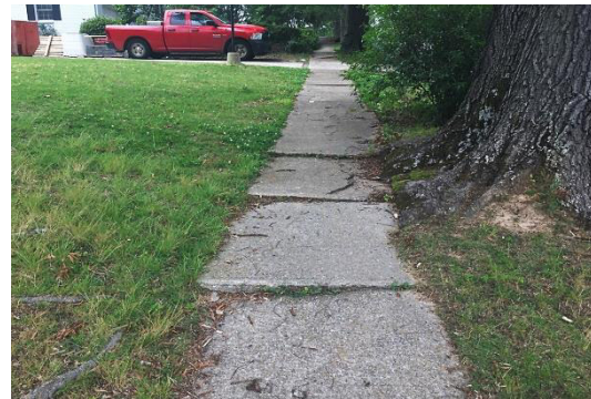
FIGURE 2: NON-COMPLIANT SIDEWALK (DUE TO CROSS SLOPES EXCEEDING 2%, SEVERE VERTICAL GAPS, AND VEGETATION PROTRUDING INTO WALKWAY)
