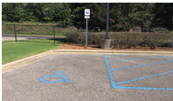
FIGURE 7: COMPLIANT ACCESSIBLE PARKING AREA
