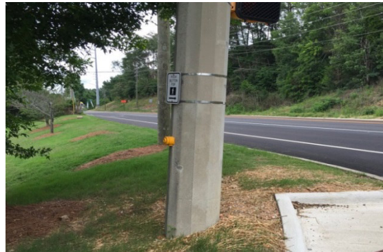
FIGURE 10: NON-COMPLIANT PEDESTRIAN SIGNAL (DUE TO EXCESSIVE HORIZONTAL REACH AND NON-COMPLIANT DISTANCE FROM CURB/PAVEMENT)
