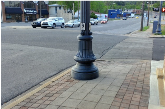
FIGURE 9: COMPLIANT PEDESTRIAN SIGNAL
