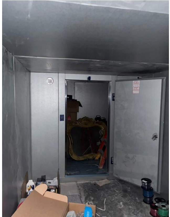
Walk-in cooler installation 2
