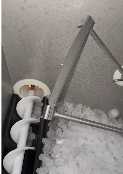
Work in progress – Inside a Hoshizaki Ice Maker Lancer bin
