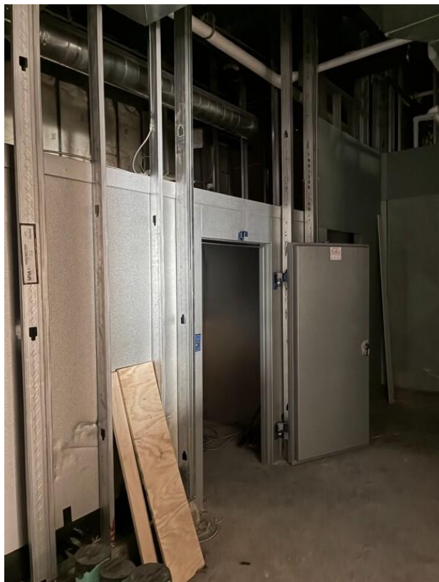
Walk-in cooler installation 3
