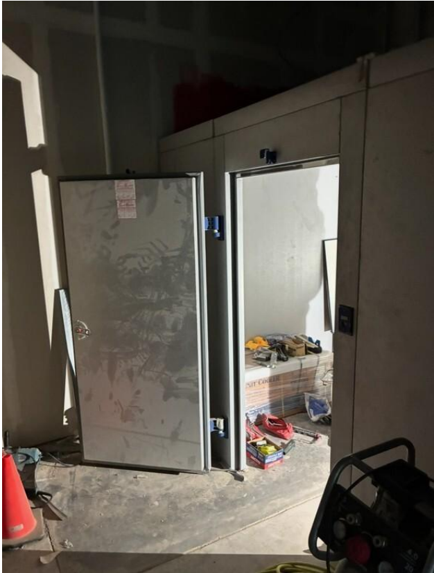
Walk-in cooler installation
