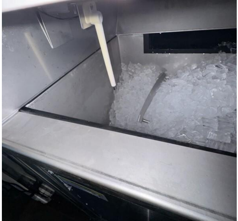
Work in progress of a Manitowoc Ice Maker bin thermostat installation
