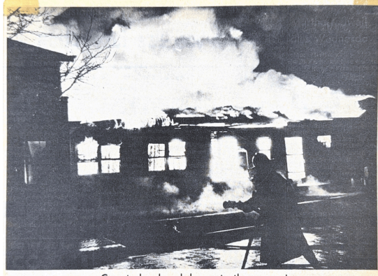
County landmark burns to the ground The Hillview Country Club building, east of Franklin on Ind. 44, a landmark structure in Johnson county for 140 years, was completely destroyed by fire late Tuesday night. Firefighters from three communities attempted to save the clubhouse. Above, flames have completely engulfed the interior of the three-story edifice and are burning through the roof. (Daily Journal photo) 1-12-71
