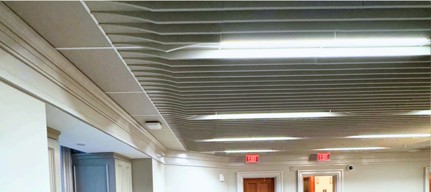
Commodore Drop in Ceiling Tiles Shown in Color Portobello (AA.85) and Tapered Edges at Perimeter
