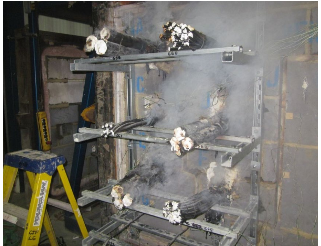
Picture shows a fire test after 2 hours at BM Trada in UK
