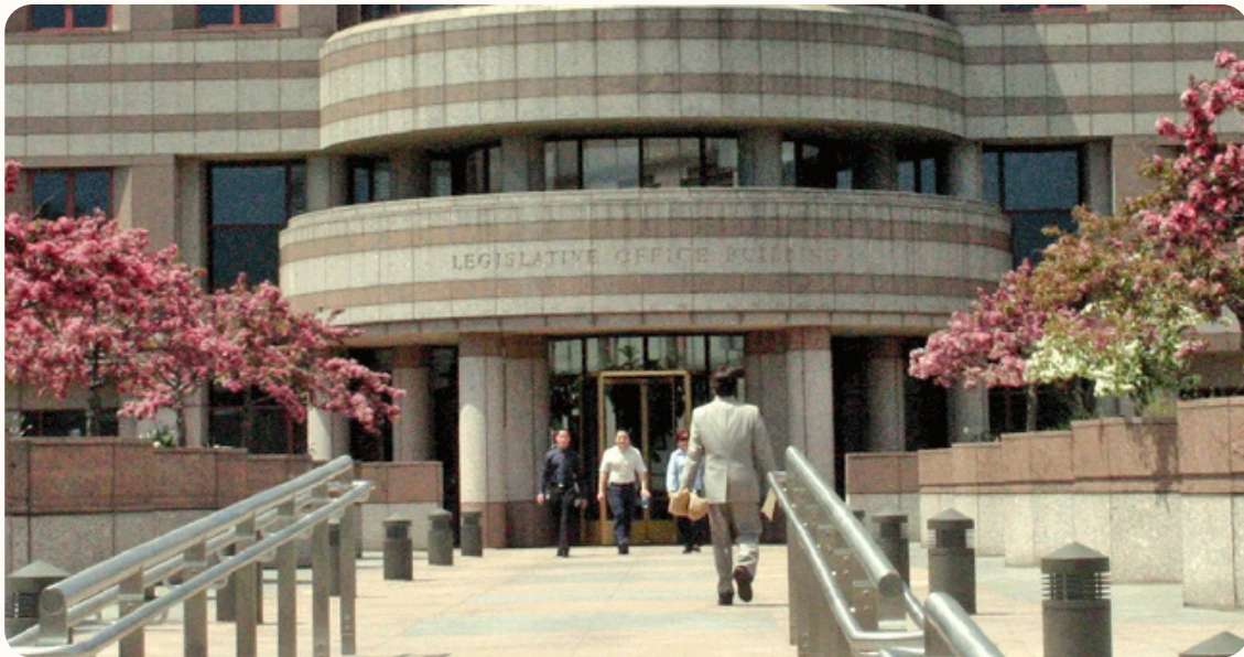
Connecticut General Assembly Building in Hartford, CT
