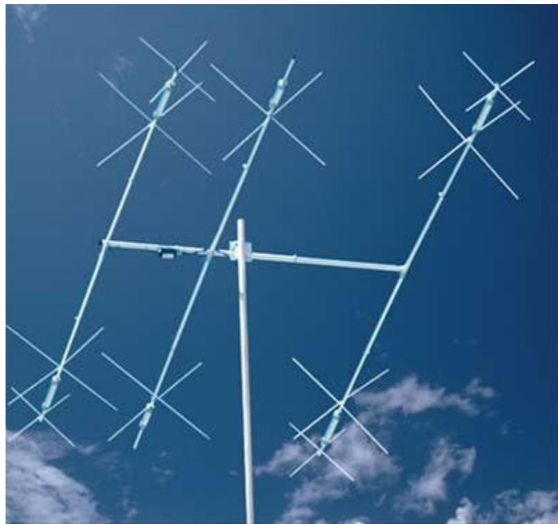
Cushcraft MA 5 multiband antenna. I have the boom and elements but still looking for a few of the capacitive hats ( the Xes) \$50
