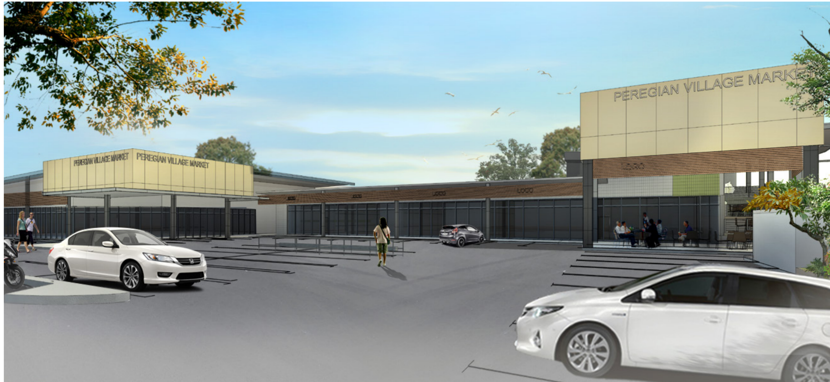
CAR PARK VIEW
