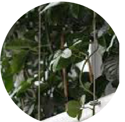
Trellis green wall system
