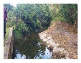
20) Cluster 4 at fifteen south- pipe is allowing silt into drain and baffle needs to be installed.
