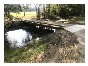
Photo below is a culvert with headwalls on the cart path roughly mid-way between holes 5 and 6 and was not previously in the report.
