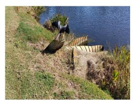
24) South course sixth hole fairway behind Quail Forest-standing water in ditch. Repair pipe and clean ditch. Pipe is not noted on drainage plans.
