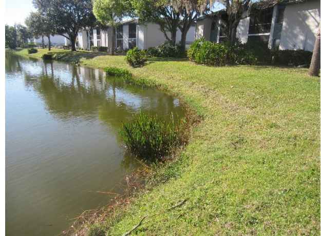
Pond shorelines – minor erosion evident
