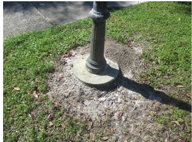
Sign and traffic signage – deterioration of the paint finishes on the post evident
