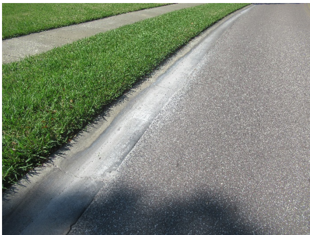
Asphalt pavement – Woodlands Drive – sediment in the gutters evident
