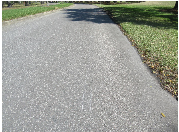
Asphalt pavement – replaced in 2012 – deterioration of the striping evident
