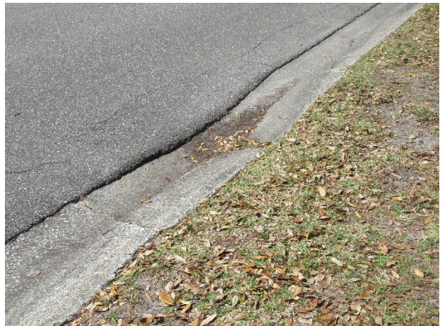
Asphalt pavement – replaced in 2011 - settlement evident
