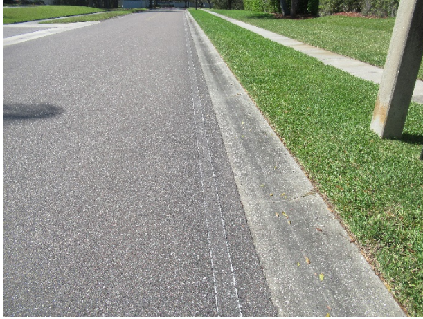
Asphalt pavement – replaced in 2011 – deterioration of the striping evident
