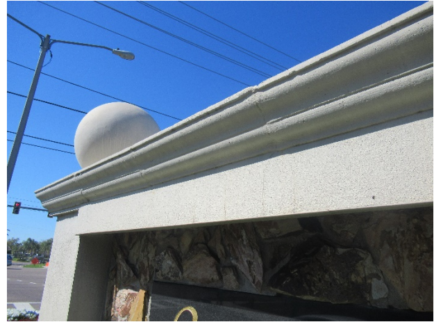
Entrance monument signage – deterioration of the top cap evident – north gate house
