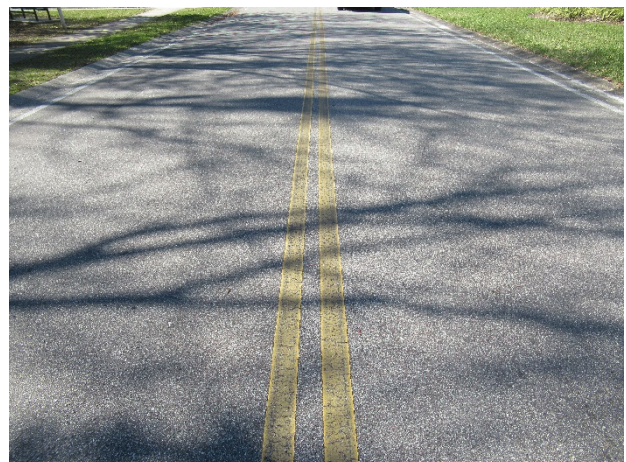
Asphalt pavement – replaced in 2016 – deterioration of the striping evident
