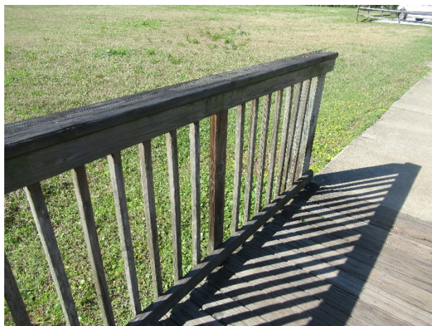
Wood walkways – partial replacements of the wood evident
