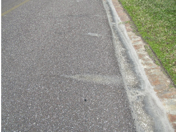
Concrete curbs and gutters – rust stains evident
