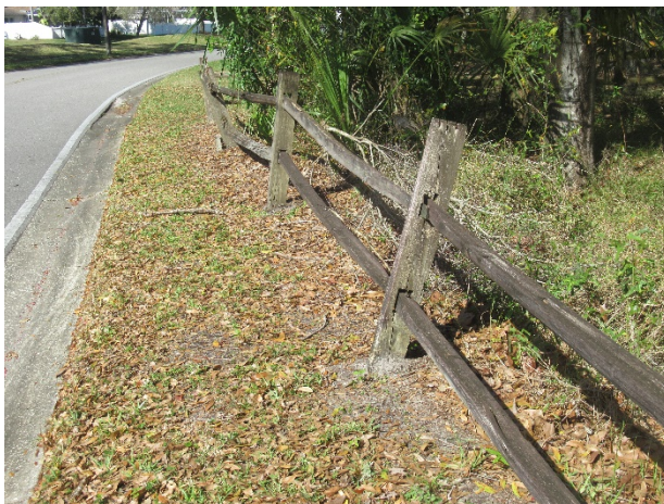
Split rail wood fences – leaning sections evident
