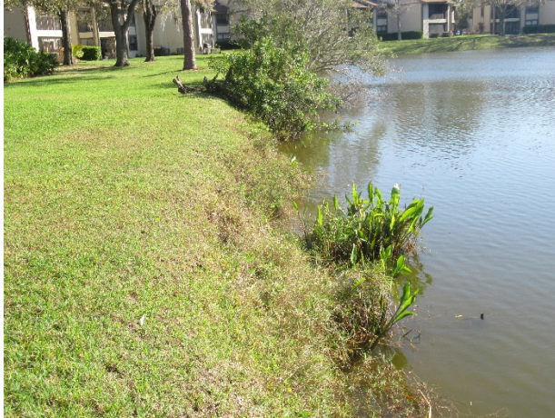
Pond shorelines – minor erosion evident
