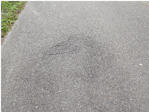
Asphalt pavement – replaced in 2008 – slippage cracks evident
