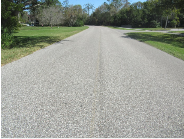
Asphalt pavement – replaced in 2008 – raveling evident
