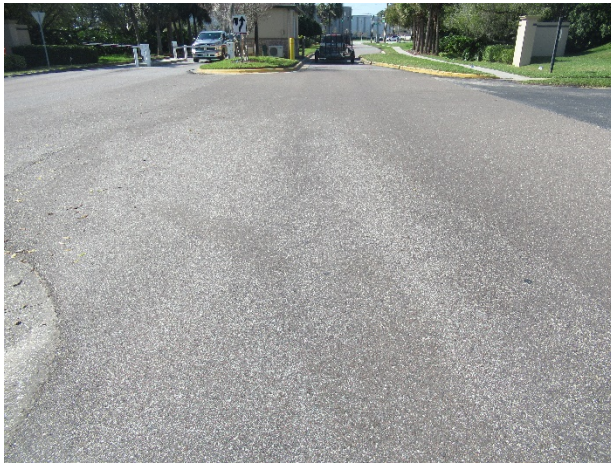
Asphalt pavement – replaced in 2012 – raveling evident
