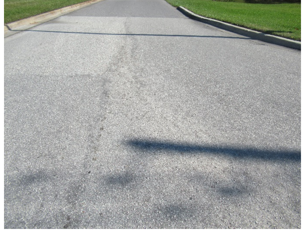
Asphalt pavement – replaced in 2012 – south gate entrance – raveling evident
