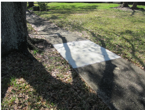
Concrete sidewalks – partial replacements evident
