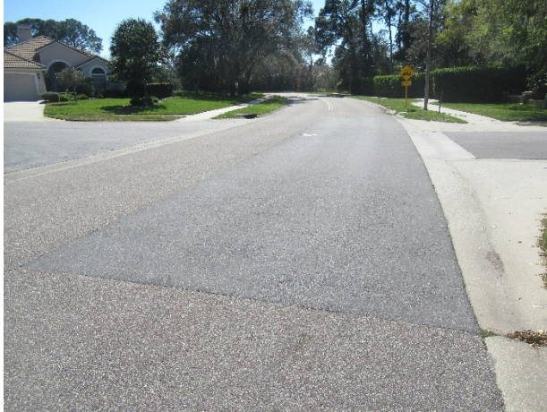
Asphalt pavement – replaced in 2013 – patch repairs evident
