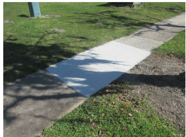
Concrete sidewalks – partial replacements evident
