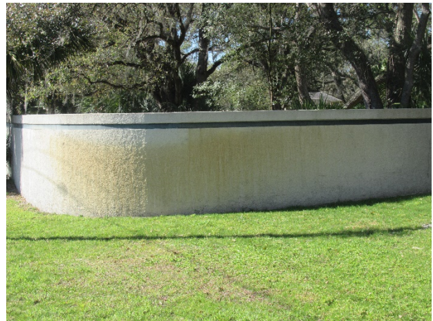
Perimeter walls – deterioration of the paint finishes evident - Sunflower
