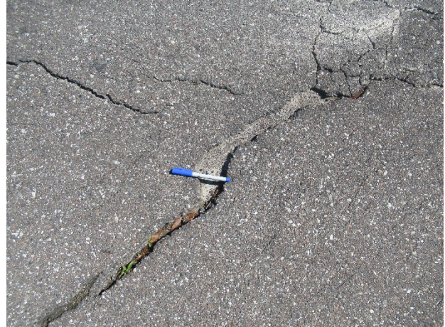
Asphalt pavement – Woodlands Drive – longitudinal cracks evident
