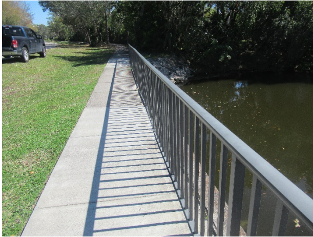
Metal railings – deterioration of the paint finishes evident
