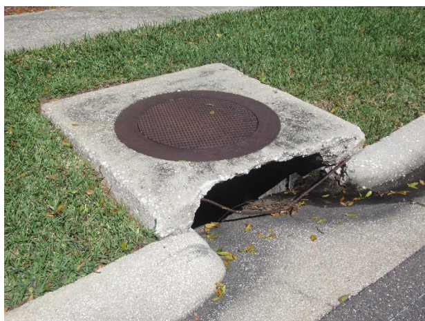
Catch basins – damaged concrete and exposed rebar evident
