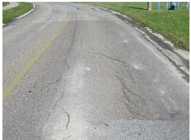
Asphalt pavement – Woodlands Drive – slippage cracks and base seepage evident
