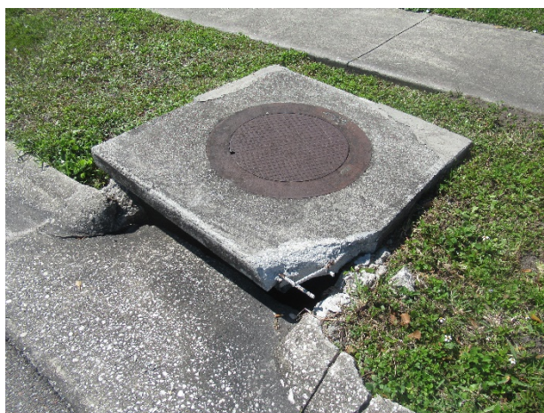
Catch basins – damaged concrete, exposed rebar, and displacement of the cap evident – near Walmart gate entrance
