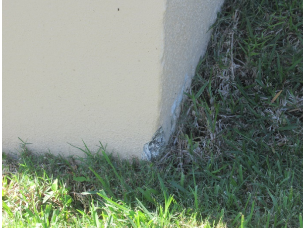
Perimeter walls – deterioration of the stucco coatings evident - South Entrance
