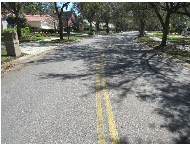
Asphalt pavement – replaced in 2015 – deterioration of the striping evident
