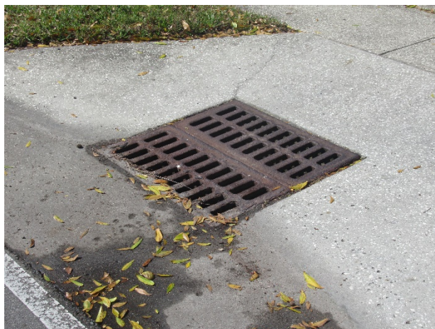
Catch basins – typical metal grated top catch basin
