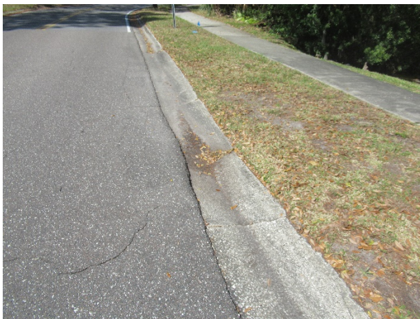
Concrete curbs and gutters – settlement evident
