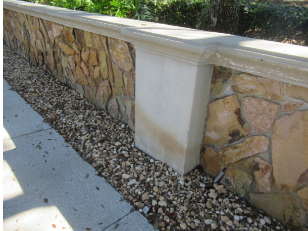
Knee walls – deterioration due to irrigation staining evident
