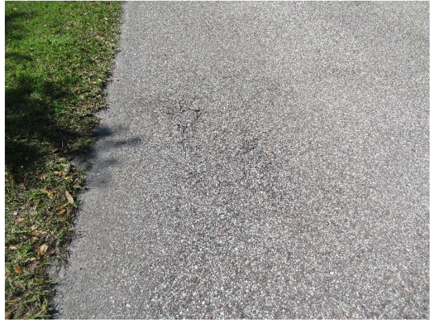
Asphalt pavement – replaced in 2008 – deterioration evident
