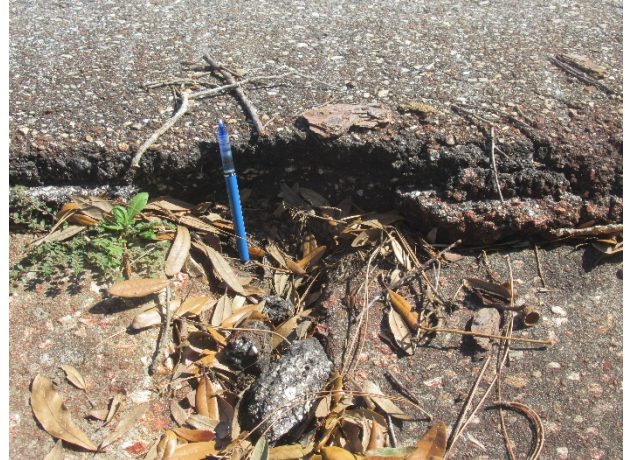
Asphalt pavement – replaced in 2013 - settlement evident at catch basin at Turtle Creek Trail
