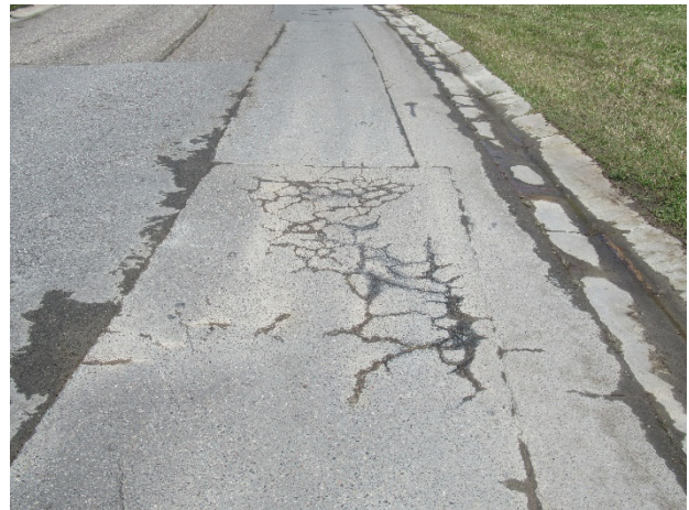
Asphalt pavement – Woodlands Drive – alligator cracks and base seepage evident
