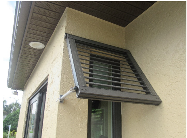
South gate house – awning and soffit
