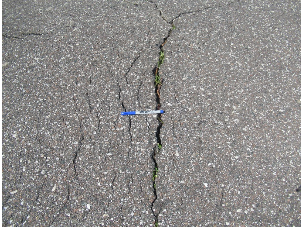
Asphalt pavement – Woodlands Drive – longitudinal cracks evident
