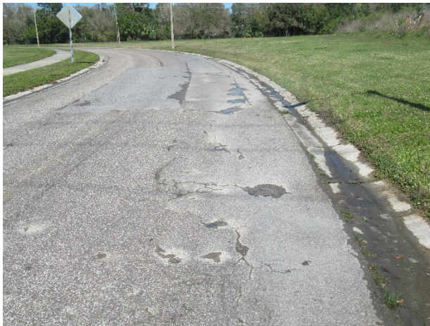
Asphalt pavement – Woodlands Drive – cracks and base seepage evident
