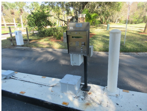
Gate entry systems – phone keypad system – Quail Forest entrance
