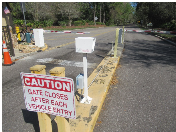
Gate entry systems – barcode scanners – East Lake Road entrance – typical scanner
