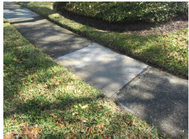
Concrete sidewalks – partial replacements evident
