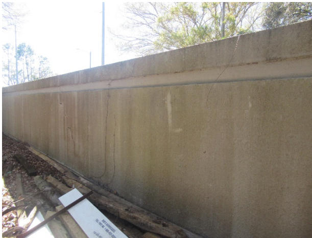
Perimeter walls – deterioration of the stucco coatings evident - Sunflower
