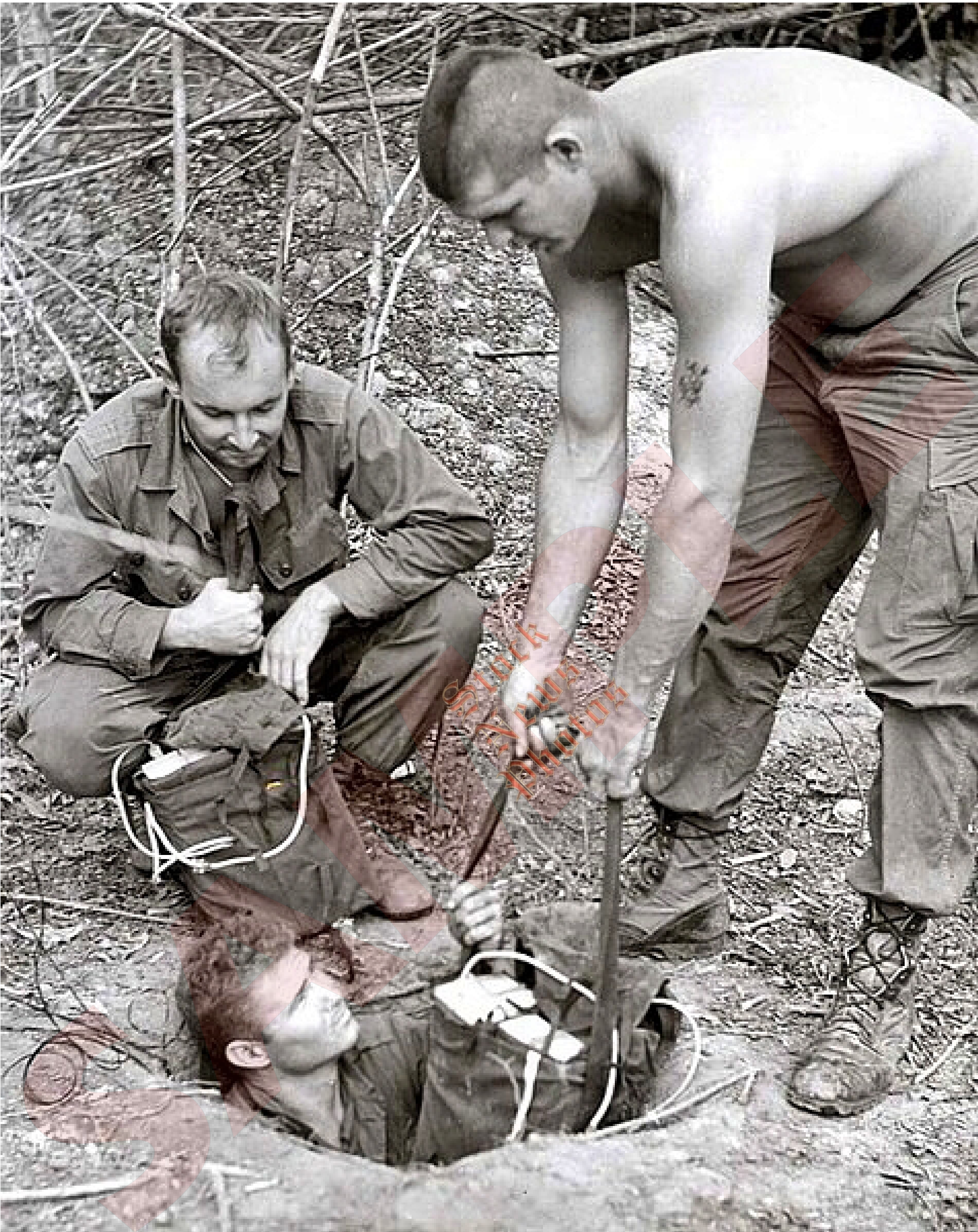
ABOVE: A Tunnel Rat can be seen preparing to enter an enemy tunnel, well concealed in the bush. Part of an Engineer Tunnel Demolition Team, explosive charges are seen being lowered into the narrow opening. Photo courtesy U.S. Army.
