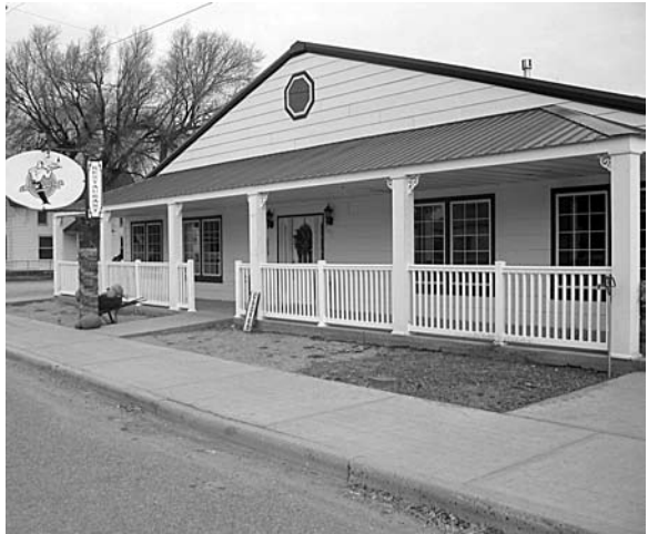
Chez W. DuVall's restaurant, Lamar, Prowers County.
