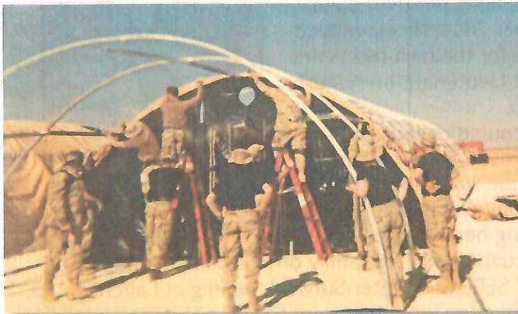
Building the hospital in Jordan January, 2003.
