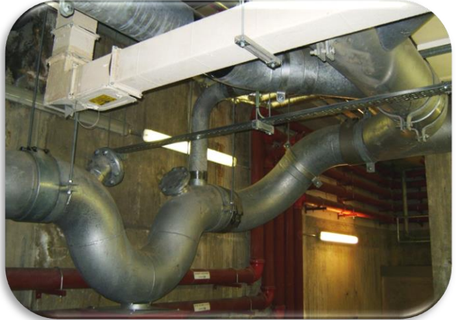
350mm,300,250 and 150mm combined drainage system
