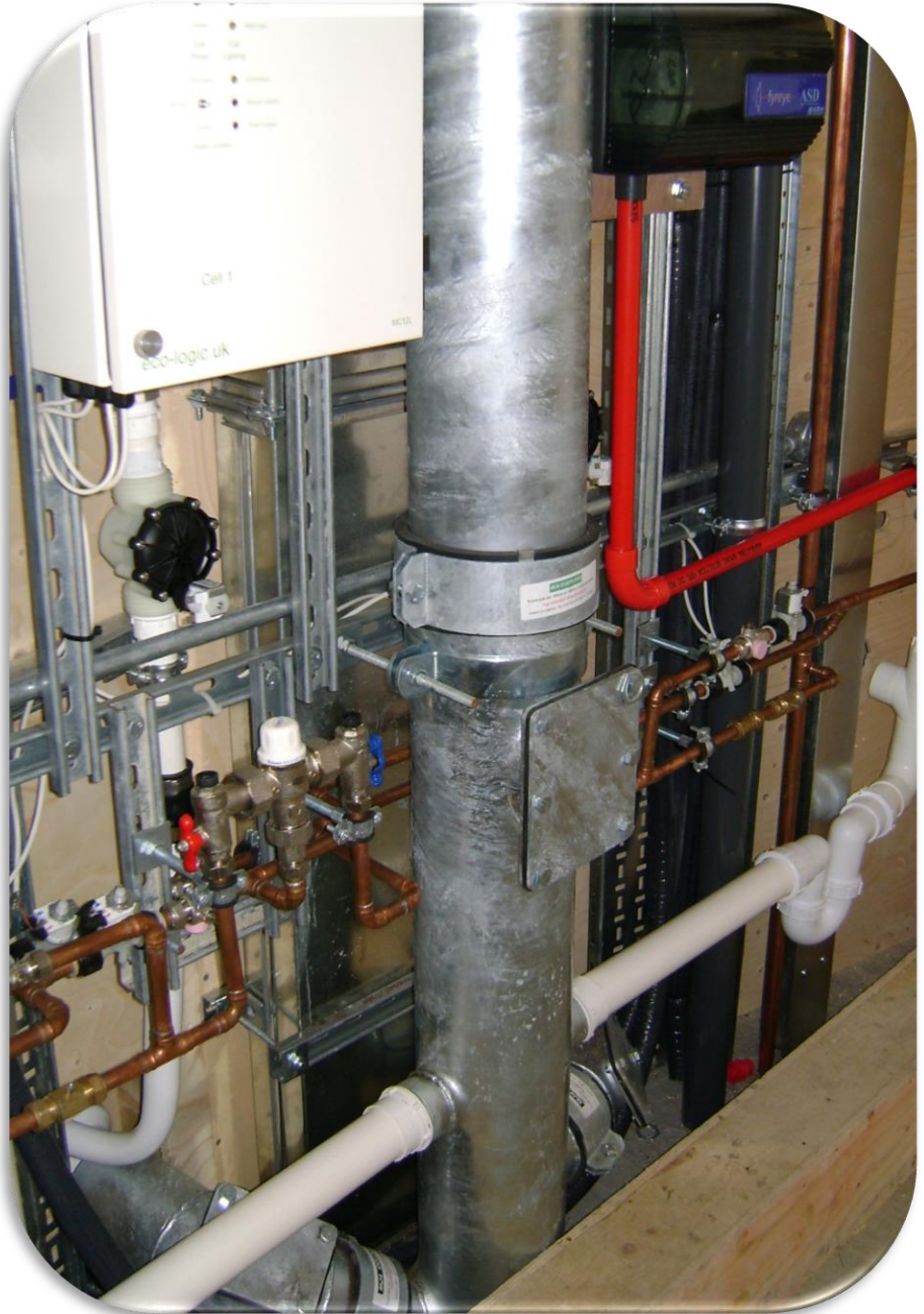
Twin Cell riser with loose pan arms. Full Roding access from all directions
