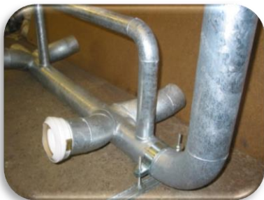
Back to back manifold with vent
