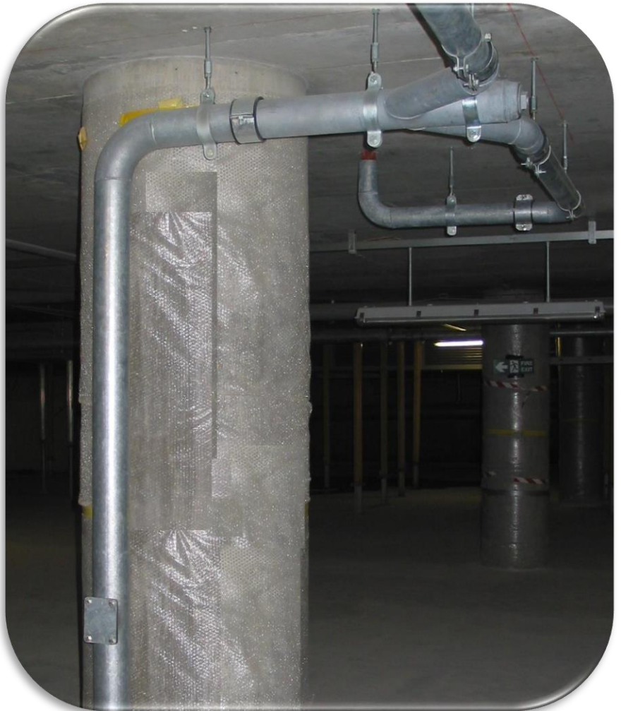
Limited joints avoids leak points caused by car damage
