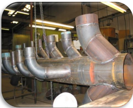
Multibranch unit being fabricated in shop
