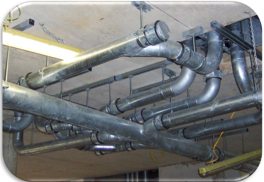
150mm and 100mm tight under slab to achieve maximum head room
