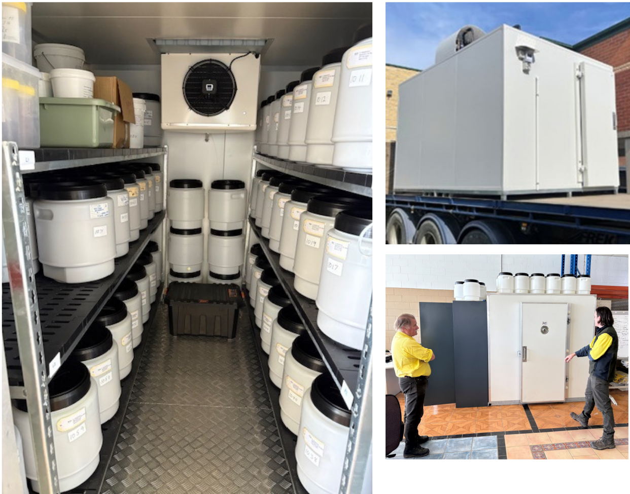
Figure 11 Demountable 14 m 3 cool room (3°C) facility commissioned by Forestry Corporation, NSW. The self-contained cold store is currently situated within an existing field depot. The facility stores up to 1 t of E. delegatensis and E. fraxinoides . Note that seed is stored in airtight containers [Photo: D. Mannes, Forestry Corporation]
