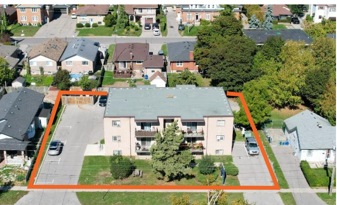
70 Orchard View, Oshawa | 12 Units
