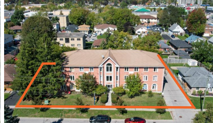
36 Orchard View, Oshawa | 12 Units
