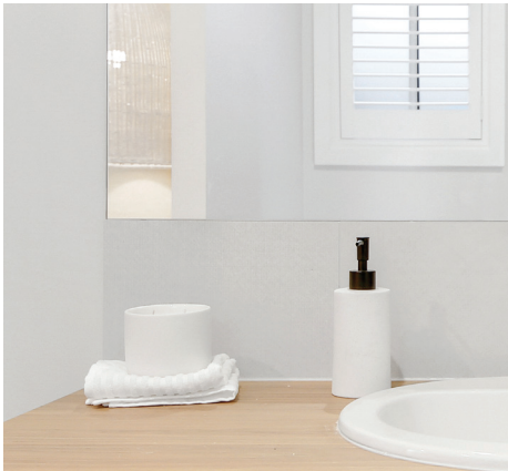
Tiled splashback Ceramic tiles to vanity splash back to 200mm high.
