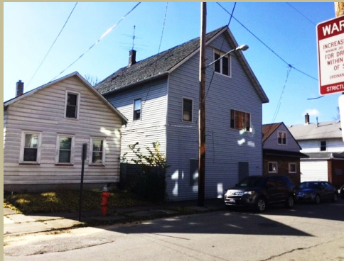
Half of Old School prior to demolition 6524 Forman
