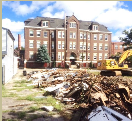
View after demolition
