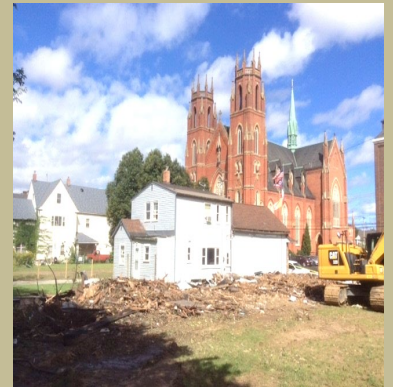
View after demolition
