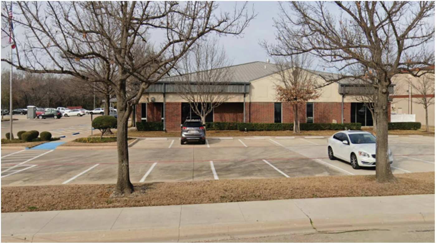
FIGURE 2.02 Front of Main Denton CAD Office Building
