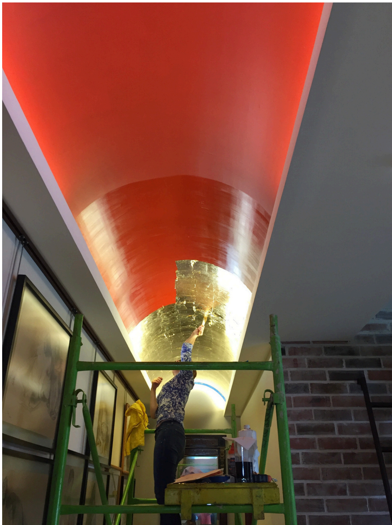
Residential Vault Gilding Gold leaf gilding 2018 In collaboration with Lupita Pedroche
