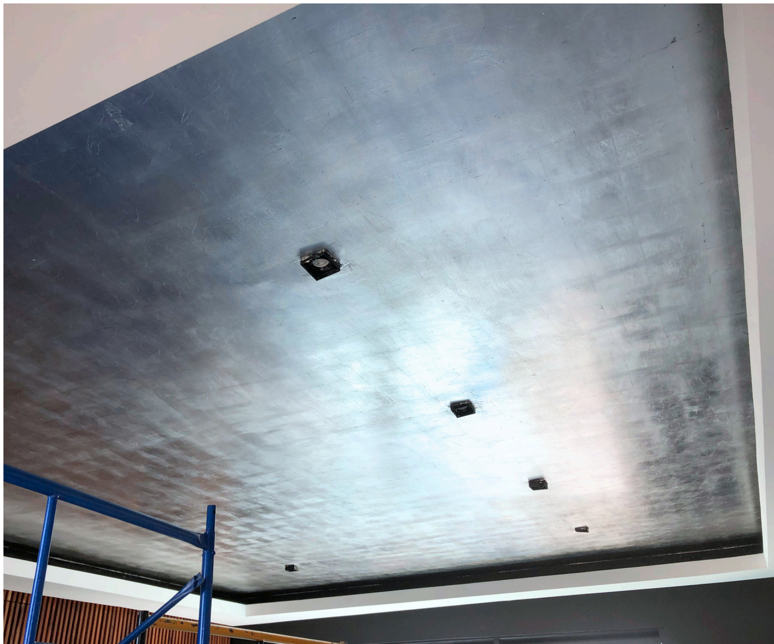
Commercial Ceiling Gilding Silver leaf gilding 2018 In collaboration with Lupita Pedroche
