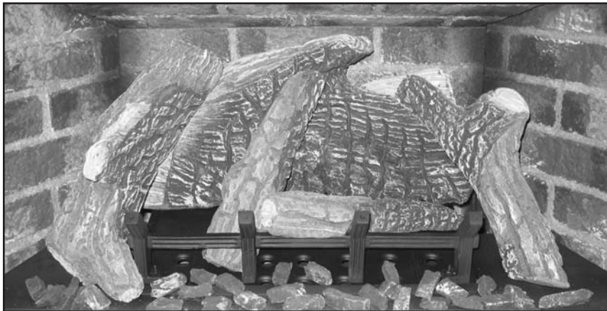
Figure 35. Fourth Stage Log Set Installation.
