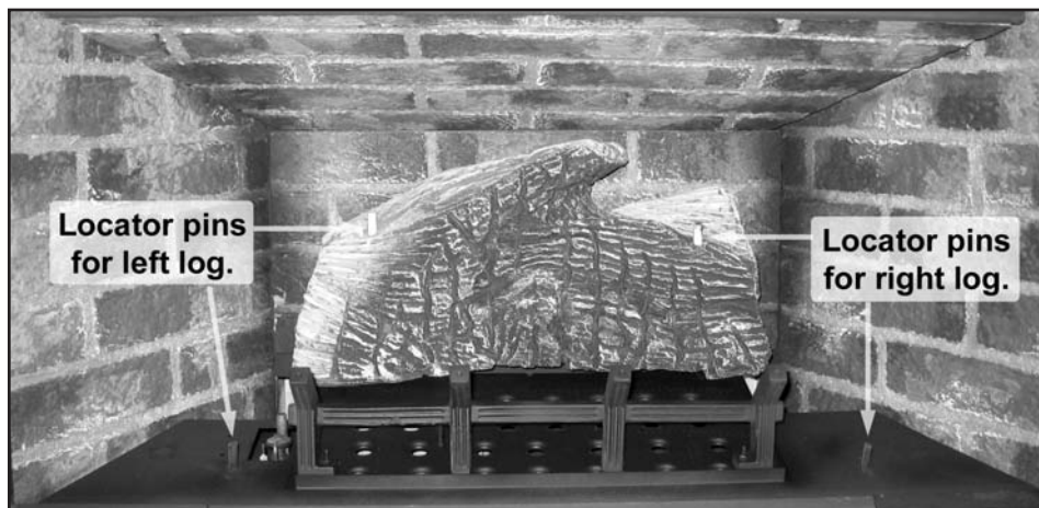
Figure 31: Empty firebox with grate and locator pins.
