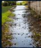
Ponding in yard after rain
