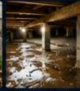
Water entering crawlspace
