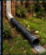
Downspouts discharge away from home
