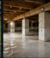
Dry, well-ventilated crawlspace
