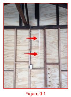
9) Wood siding is exposed to sprinklers and rain run off. This will deteriorate material over time of exposure.
