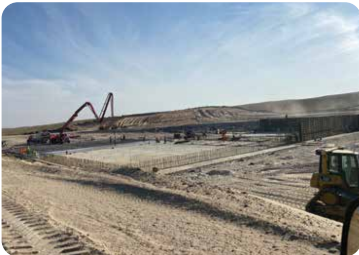
Valentine Hog Confinement Project
