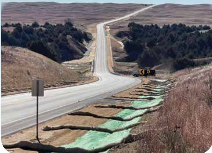
Asphalt Paving - Tryon to Mullen
