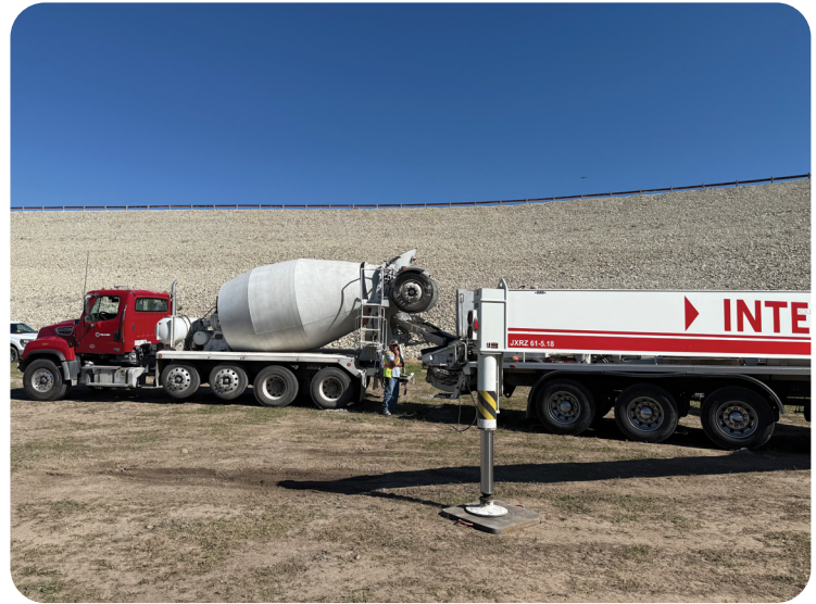
Supplying Concrete at Medicine Creek Dam
