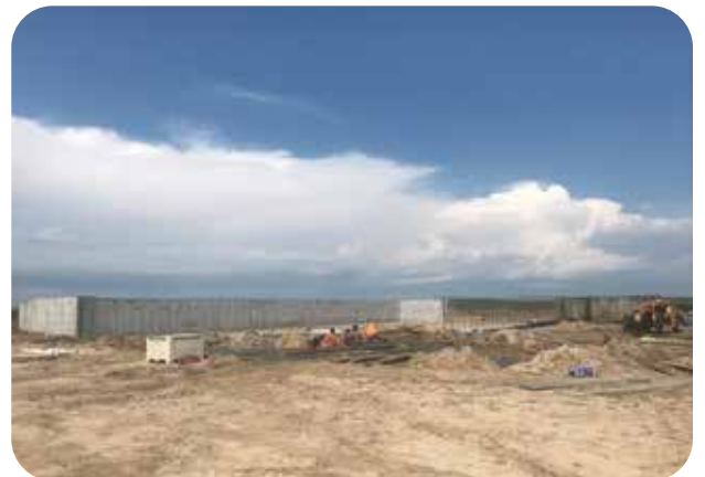
Potato storage building south of North Platte
