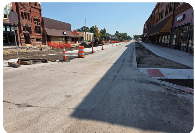
Work in Red Cloud
