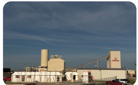
McCook Ready-Mix Plant Construction
