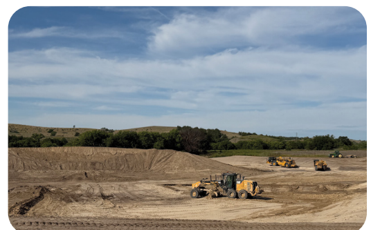
Cedar Valley Shooting Range Earthwork
