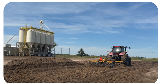
Livestock Nutrition Building Earthwork
