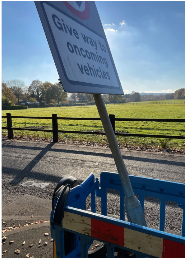
Traffic calming in School Road is not installed to standard and repeatedly damaged by having been placed on a blind bend
