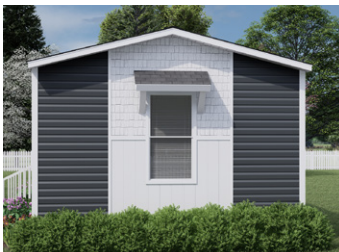
Hitch End Elevation with Shed Roof, Shakes/Board & Batten and Window Trim
