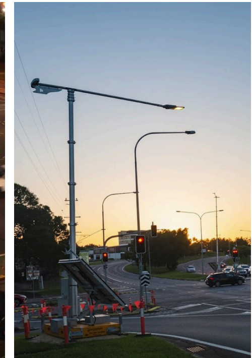
Large Intersection achieved compliant lighting using on 4 x Hammer Head units with 12m Mounting Height and Type 4 Optics
