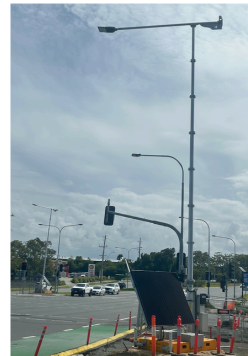
Large Intersection achieved compliant lighting using on 4 x Hammer Head units with 12m Mounting Height and Type 4 Optics
