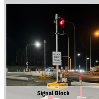
Signal Block Temporary signaling units for traffic management
