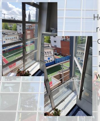
Here we have a window we repaired In The HSE head office. This window could not be opened when we arrived. Due to Covid 19 we had to get the window open and replace the hinges allowing airflow through the building.
