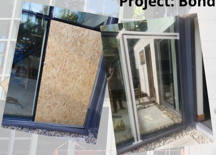
Here we boarded up a broken window and replaced the glass and re bonded the curtain walling on this emergency job
