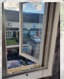
To the left is a sash that we fitted fire escape hinges to to allow the window to open 90 degrees to allow fire escape from upstairs.
