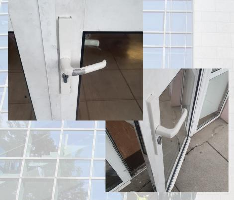
On this job we were required to replace door handles to an isolation wing that had been damaged.
