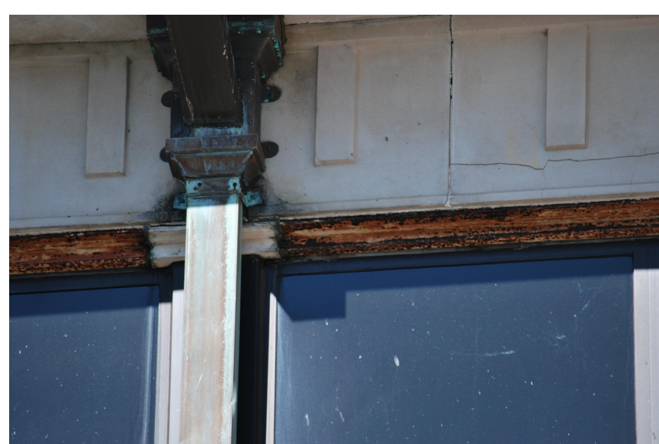
A3 ALT NO. 3 CAST STONE FRIEZE REPLACEMENT
