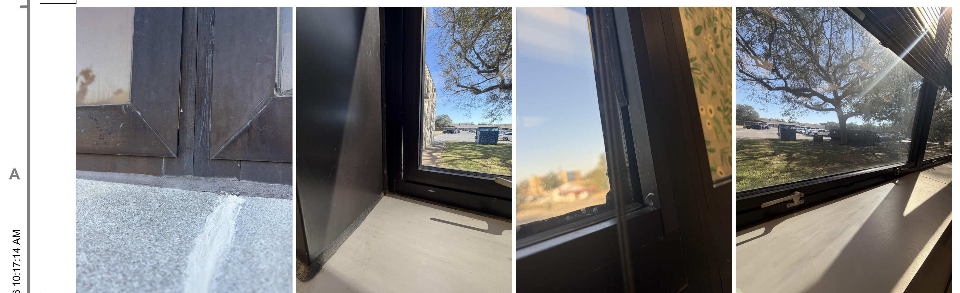
A1 OPERABLE SASH REFERENCE PHOTOS SCALE: 3/4" = 1'-0"
