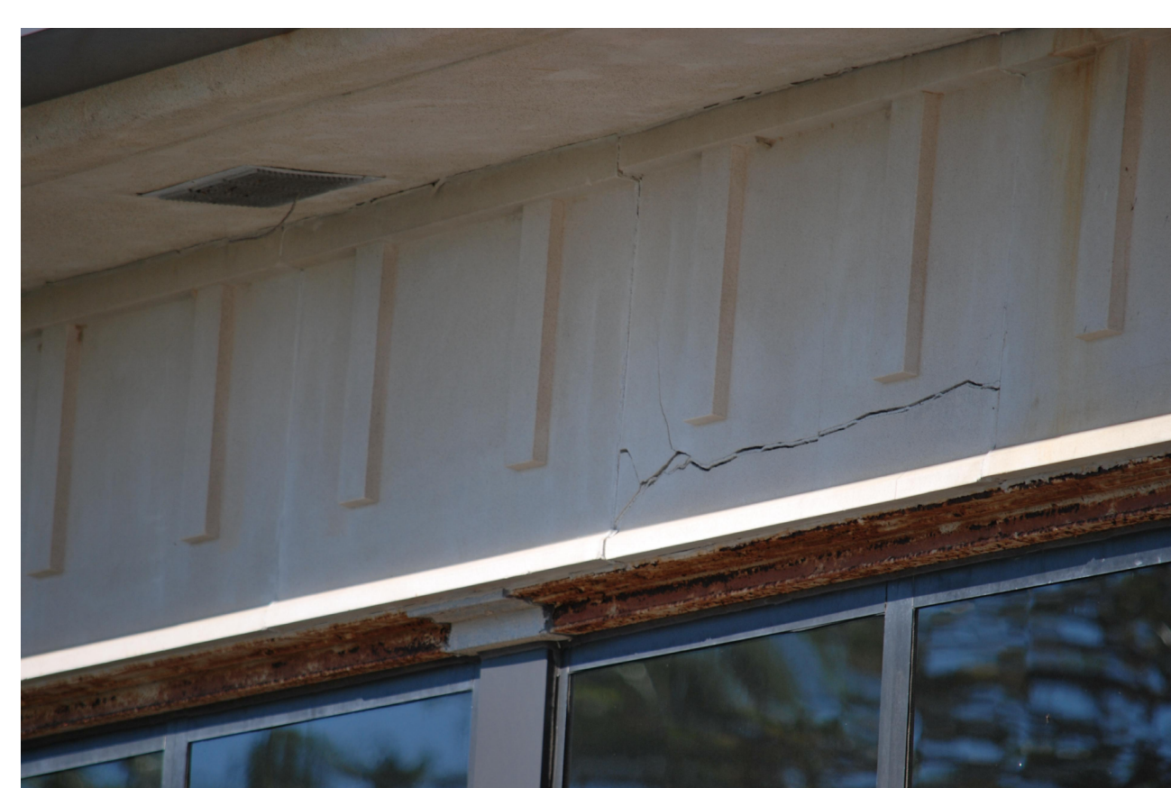
A2 ALT NO. 3 CAST STONE FRIEZE REPLACEMENT
