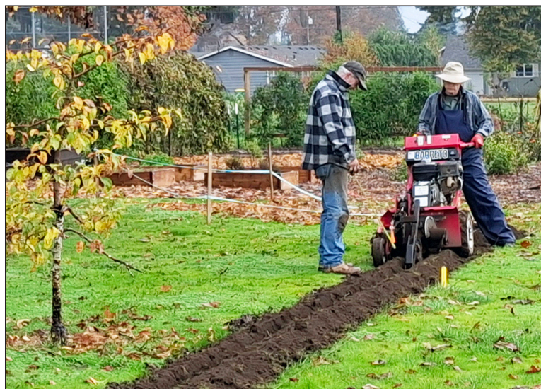
Charlie Rhyne (left) and Scott Richards (right) use rented trencher to install efficient irrigation system, late fall 2025.
