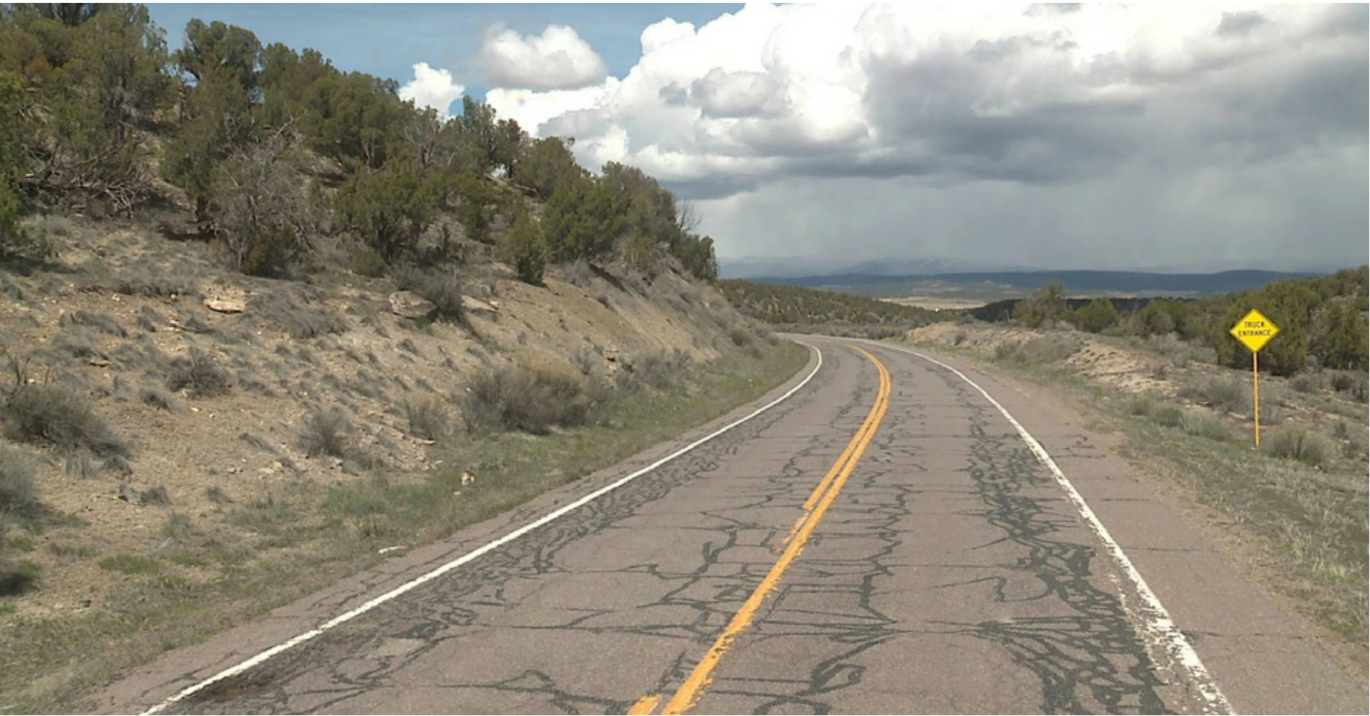
Poor pavement along a rural state highway
