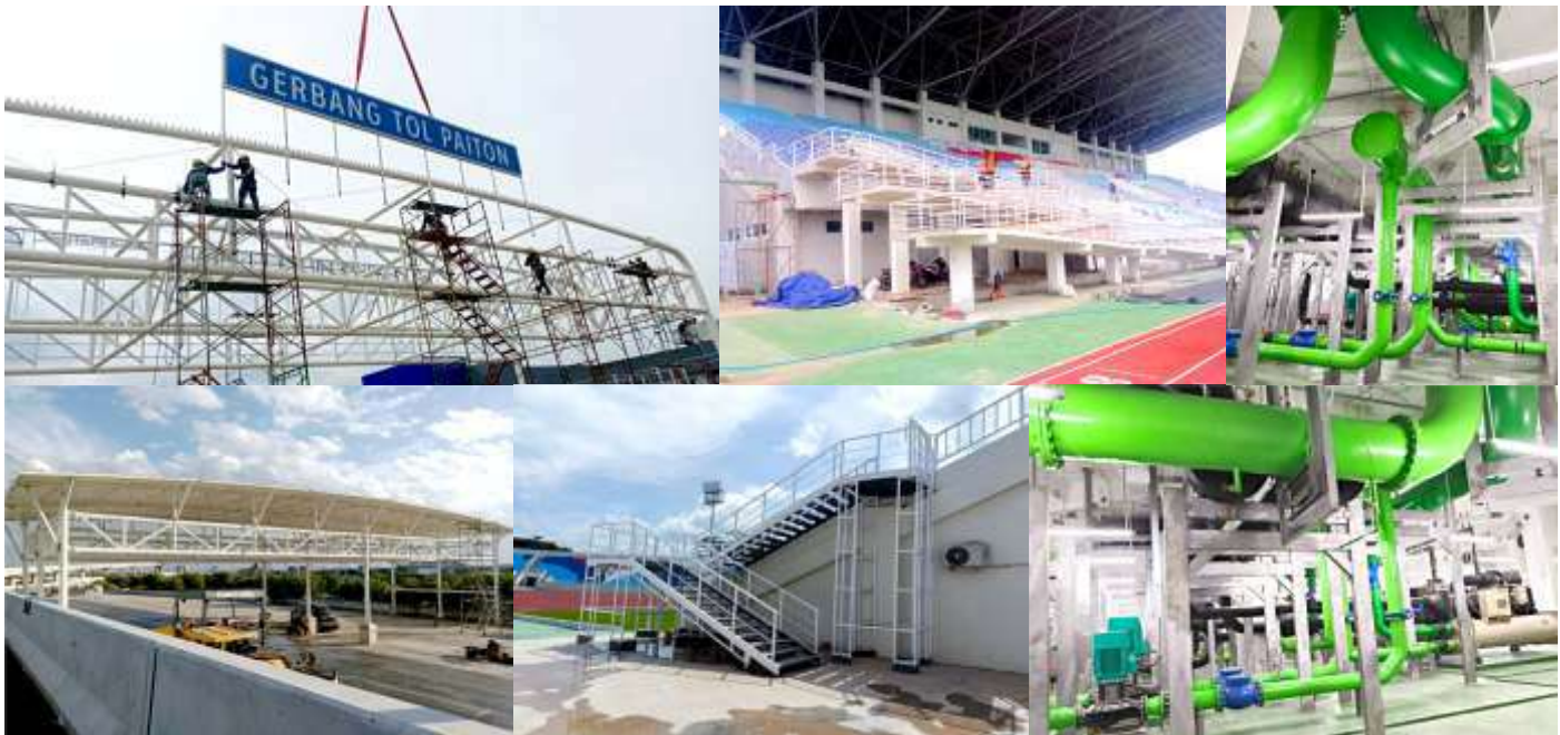
[07] Revitalisasi Dermaga Gospier Surabaya | [08] SPAM Jatiluhur | [09] Proyek Dermaga Batu Bara – PT Pupuk KalTim [10] Project Dermaga Tanjung Wangi (Tambahan) | [11] SPAM Jatiluhur | [12] Proyek Dermaga Batu Bara – PT Pupuk KalTim
