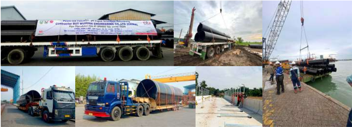
[01] Pipeline IAE Gresik | [02] Dermaga FT Luwuk & FT Raha di Sulawesi Tenggara | [03] Batu Hijau Expansion Project [04] JAB Bendungan Paselloreng – Wajo | [05] Proyek Sumbawa Timur Mining | [06] Rehabilitasi Pelabuhan Penyeberangan Pananaru
