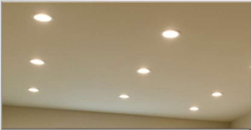
Dimmable Recessed Lighting for Ambient Light (qty 11)
